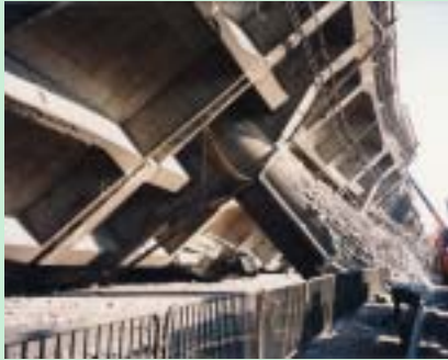
Collapsed single pier elevated highway bridge due to the 1995 Kobe earthquake
