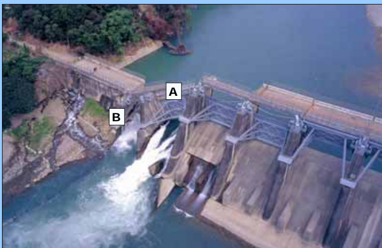
Figure 5 damage just above the fault
