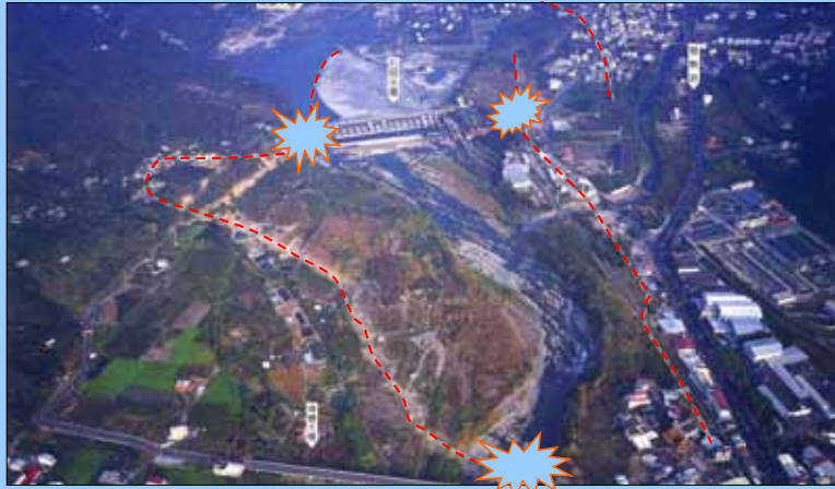
Figure 1. Damage on the infrastructure in the Shih-Kang area [1]
