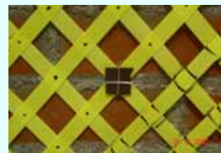
6. Detail of wire connectors through the wall
