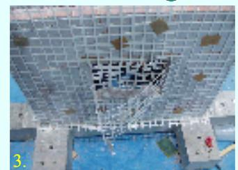
3. Connecting inner and outer meshes by wires and aluminum plates (2cmx2cm) except around the openings.
