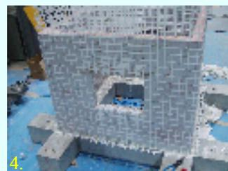
4. Fixing connectors around the openings after the mesh is cut and overlapped on the other side.
