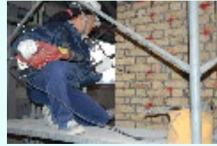
1. Drilling holes on wall
