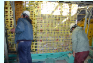
3. PP-band mesh is wrapping around openings and fixed by connectors
