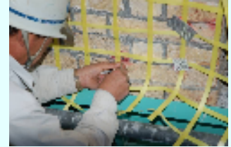
2. Connecting inner and outer meshes by wires and aluminum plates
